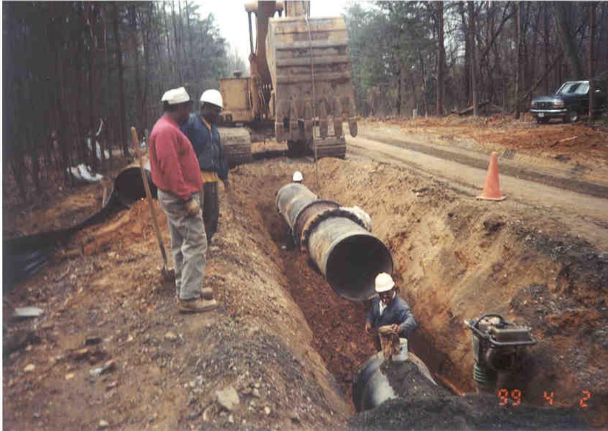
Figure 6. Traditional “Open-Cut” Piping Installation in a Roadway Shoulder
