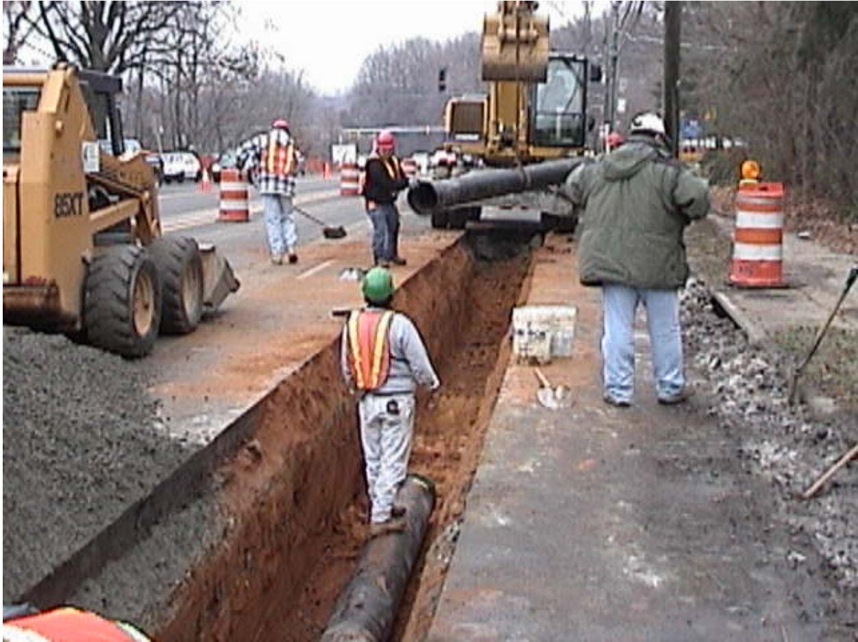
Figure 5: Traditional “Open-Cut” Piping Installation in a Road
