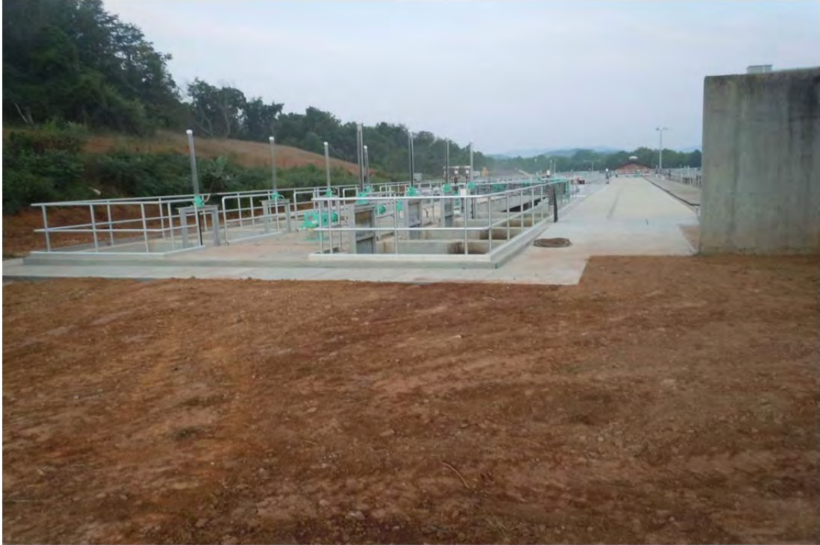
Grading near Flow Distribution Box and Aeration Basins
