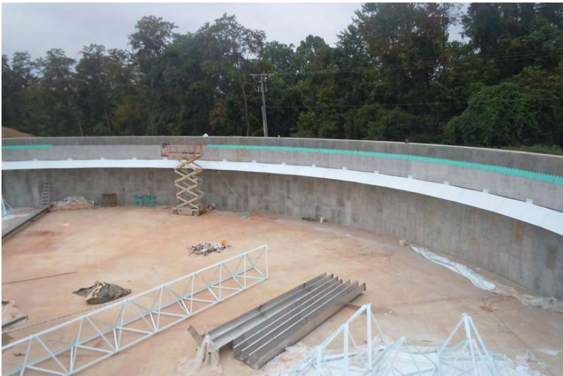
Installation of Weirs in Secondary Clarifier No. 3
