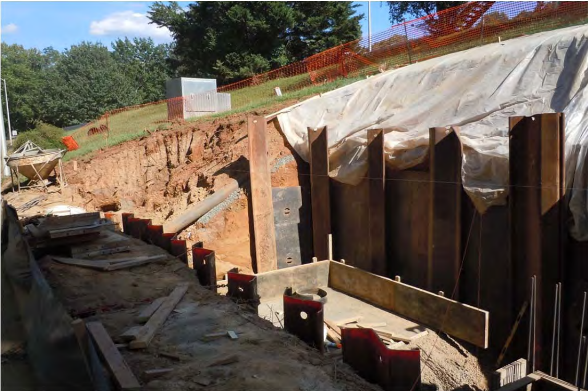
Force Main to Holding Ponds Meter Vault Construction
