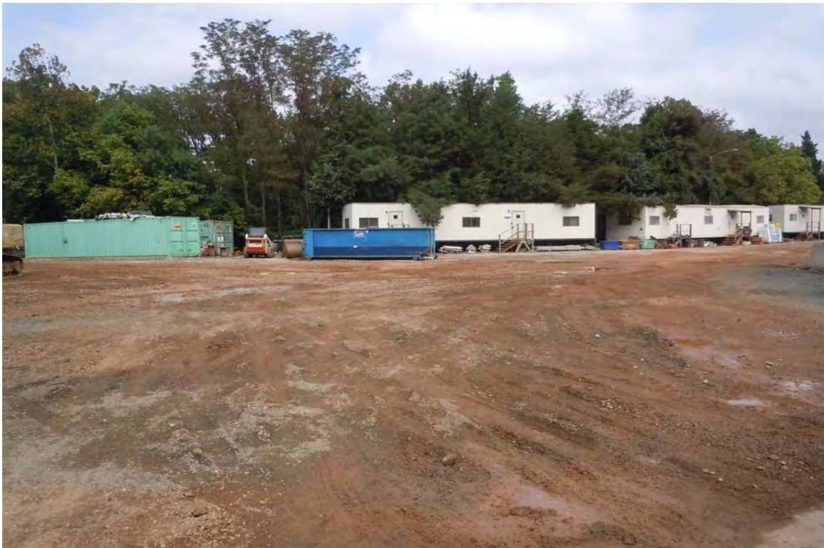
Maintenance Parking Lot – Extensive Excavation and Pipe Installation
