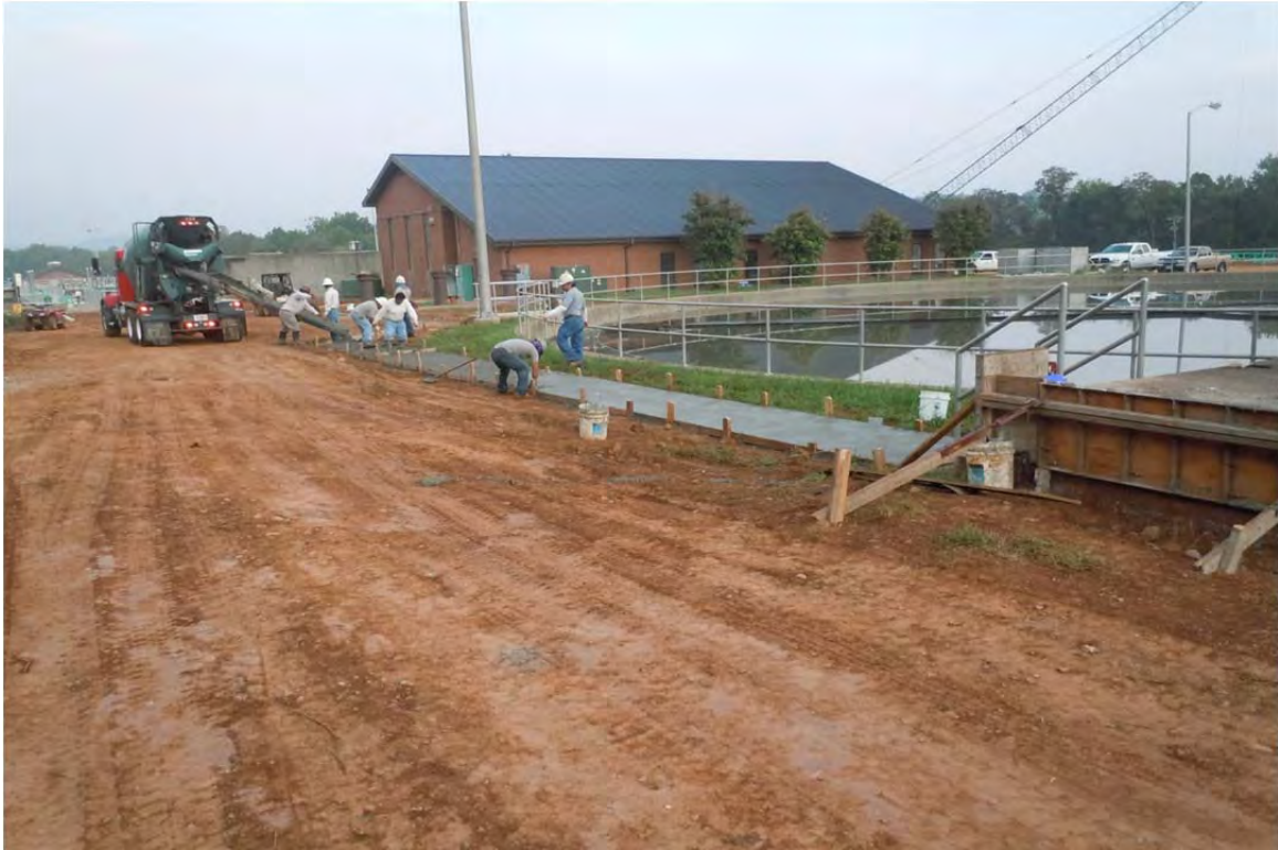
Grading and Sidewalk Construction near Primary Clarifiers
