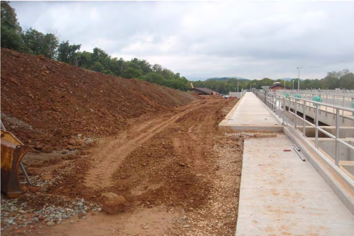
Grading on South Side of Aeration Basin No. 5
