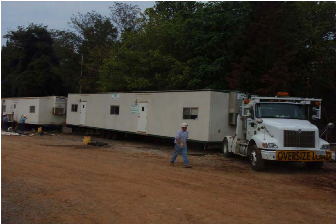
Relocation of Construction Trailers for Pipe Installation
