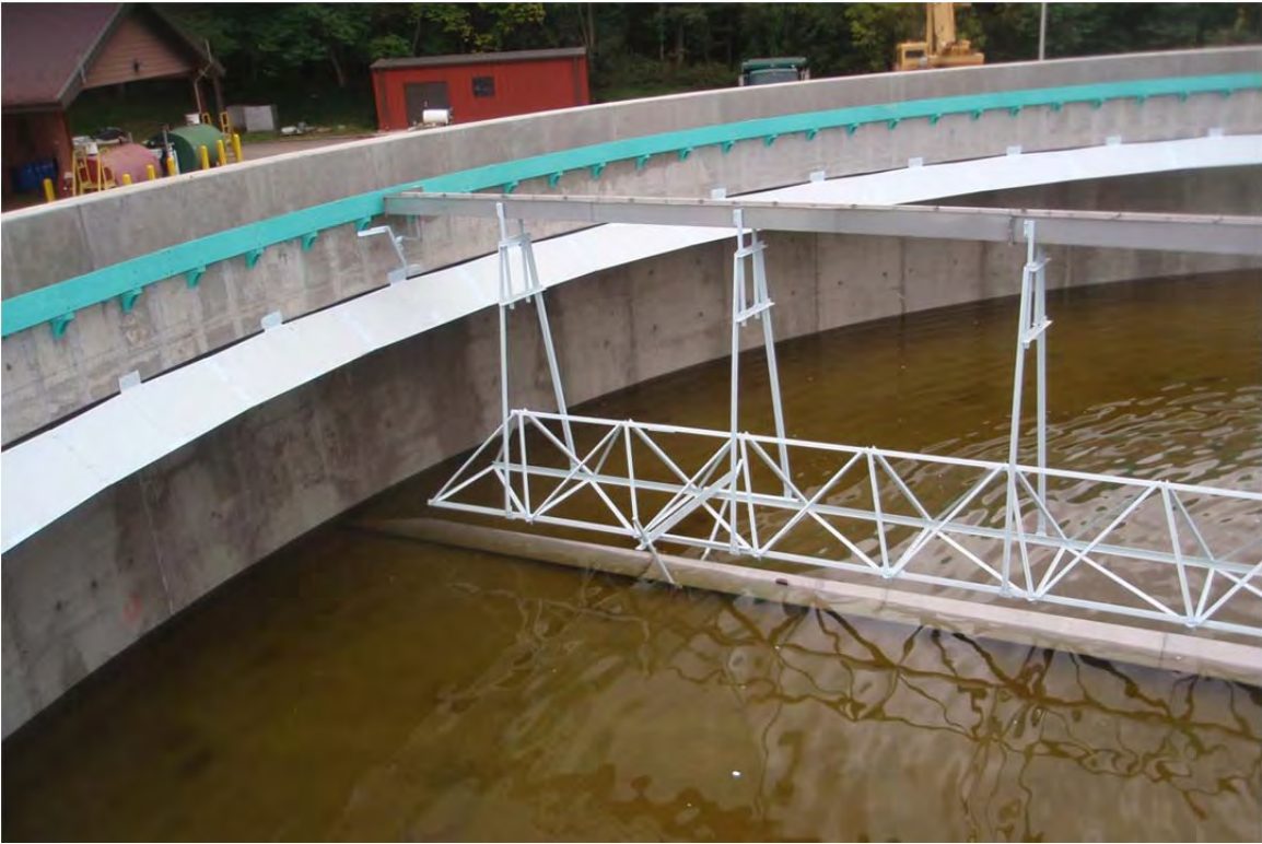
Interior of Secondary Clarifier No. 4
