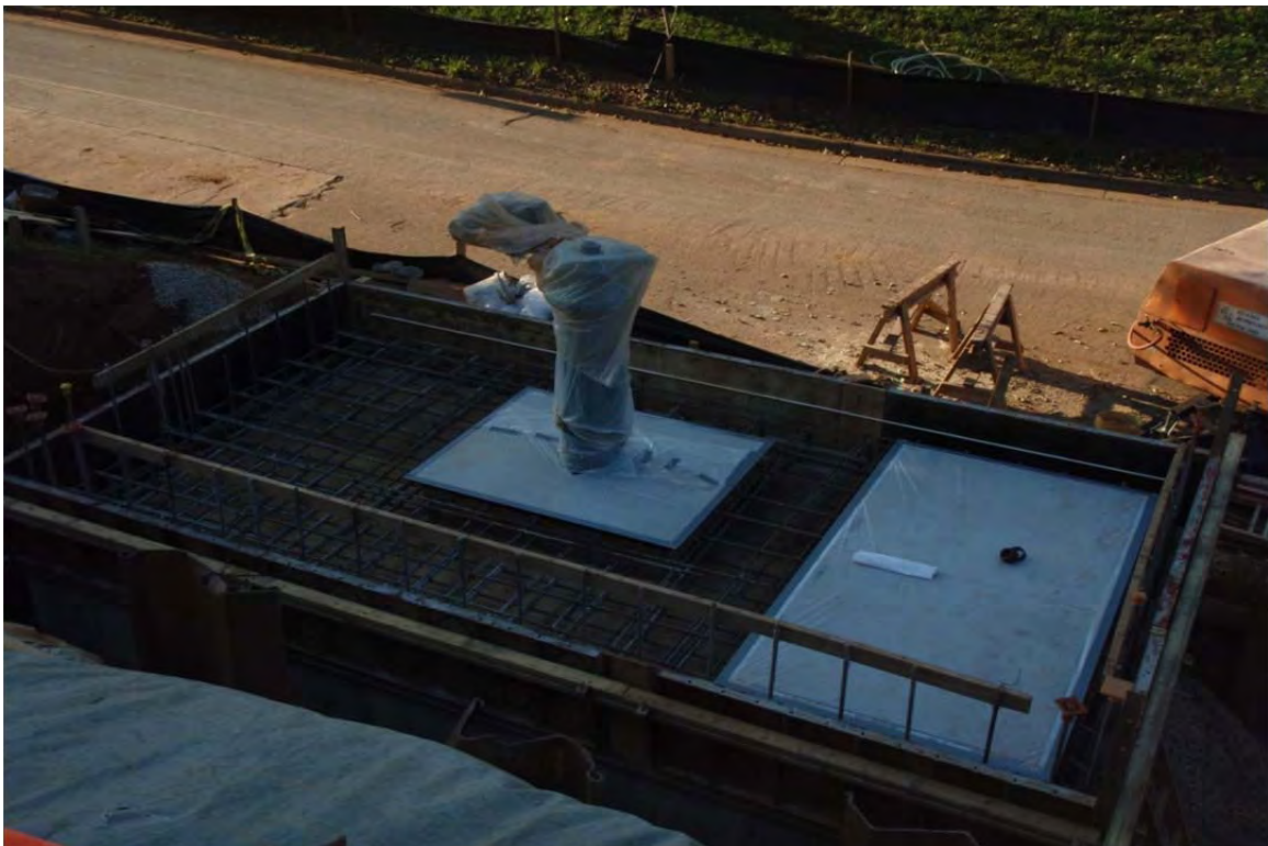
Holding Pond Force Main Metering Vault – Concrete and Steel Under Construction
