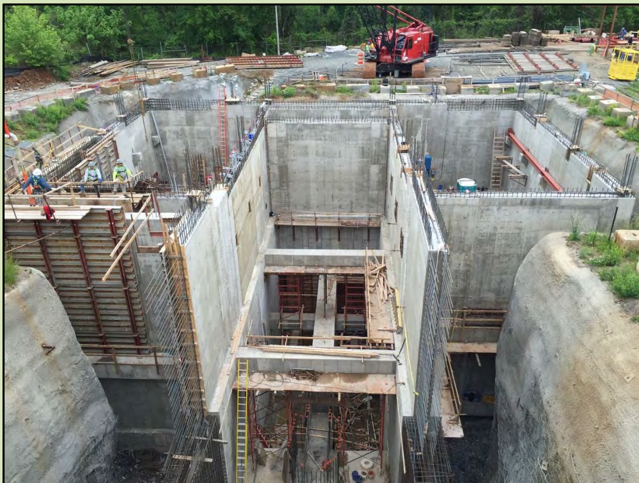
Rivanna Pump Station and Tunnel Project Charlottesville, Virginia
