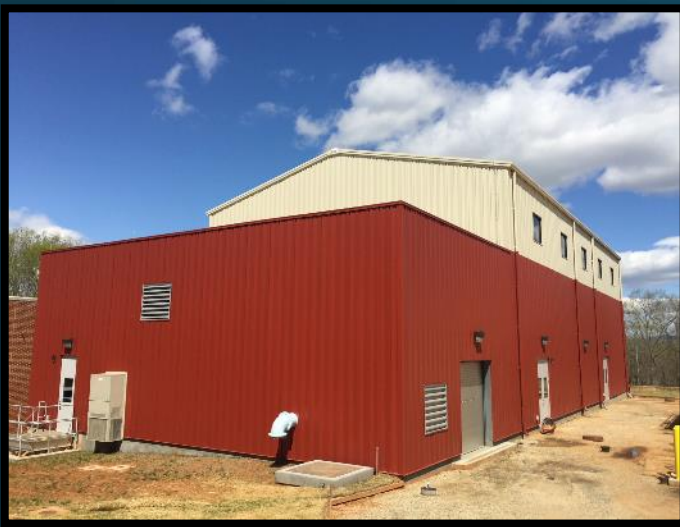
S. Rivanna WTP 8 Contactors 320,000 lbs of GAC 8 MGD Capacity
