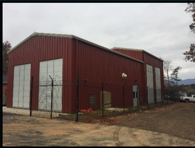
Crozet WTP 2 Contactors 40,000 lbs of GAC 1 MGD Capacity
