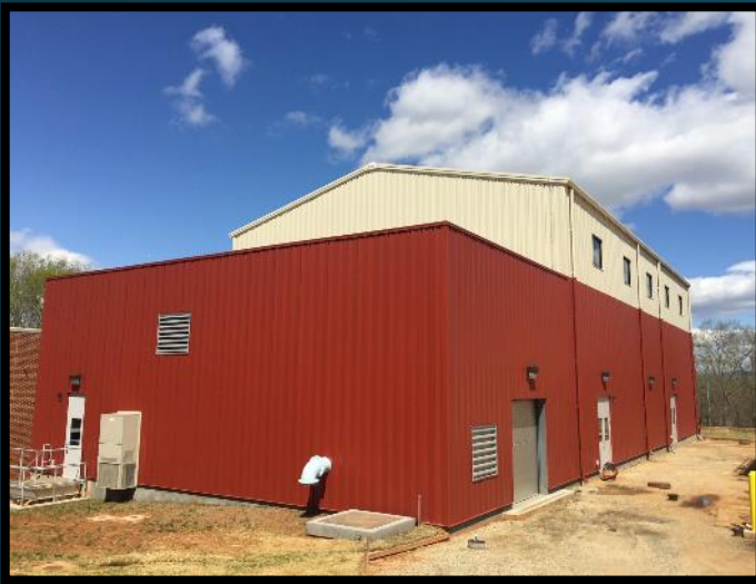
South Rivanna WTP 8 Contactors 320,000 lbs of GAC 8 MGD Capacity
