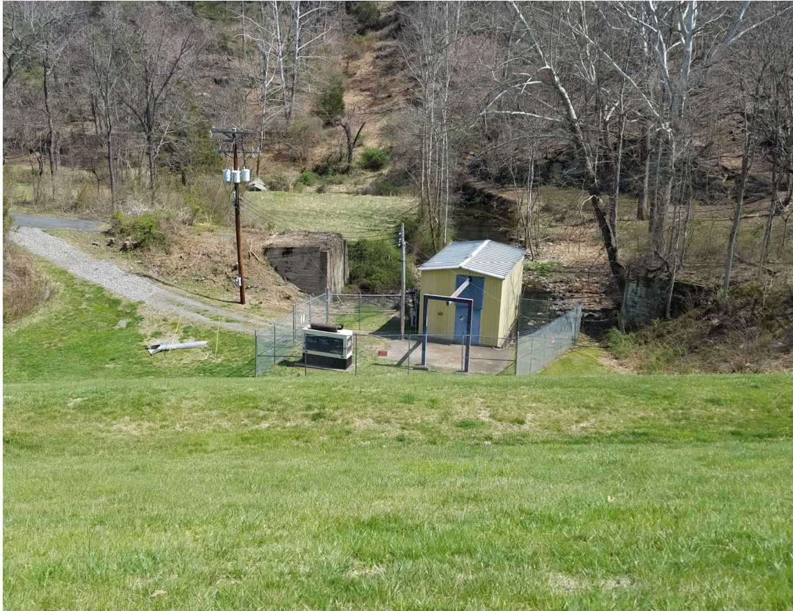
Figure 1-6: Photo of Existing Raw Water Pump Station at foot of Beaver Creek Dam
