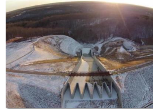
Proposed Labyrinth Spillway thru Dam with Bridge
