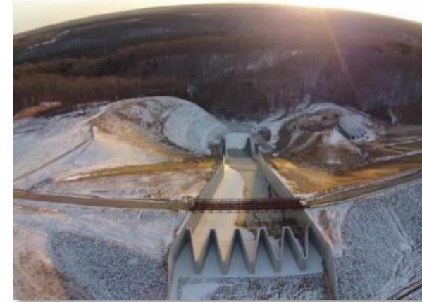
Proposed Labyrinth Spillway thru Dam with Bridge
