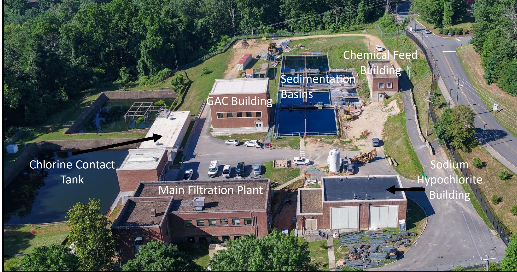
Observatory Water Treatment Plant 7.7 to 10 MGD treatment capacity
