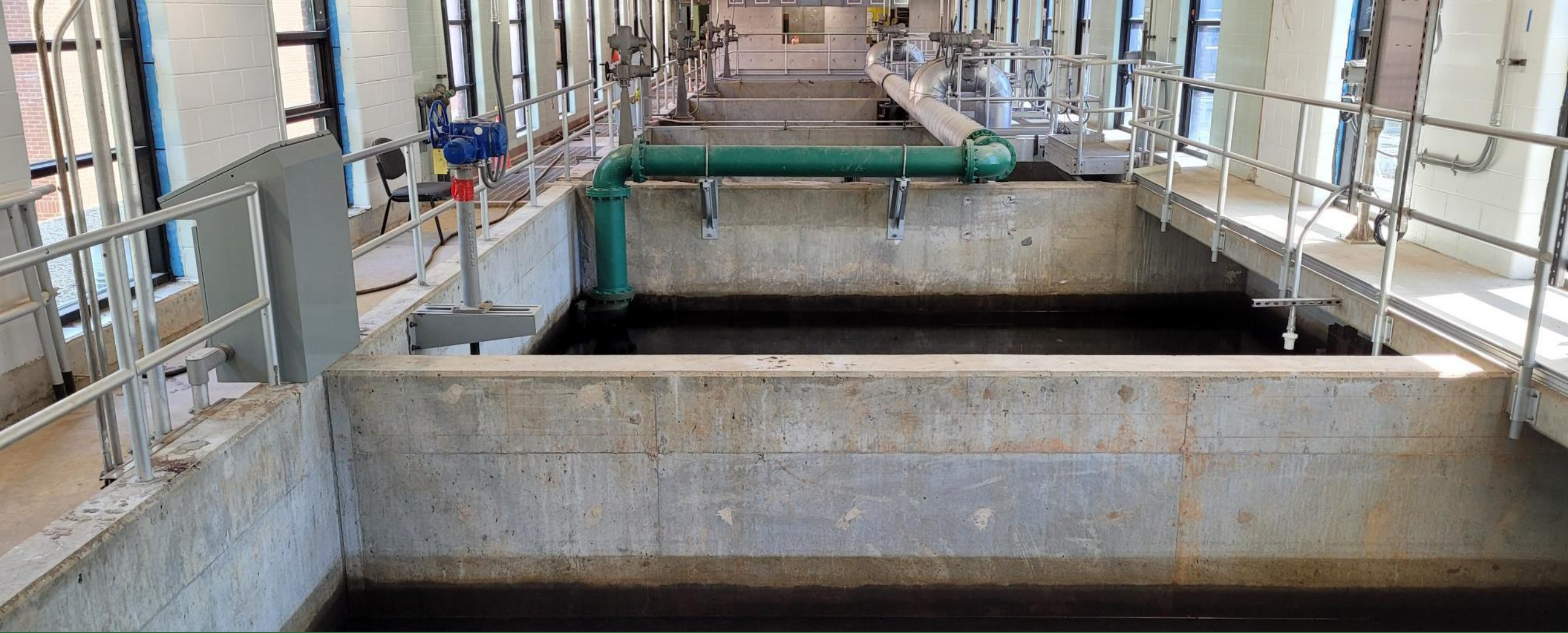
Filters at South Rivanna Water Treatment Plant
