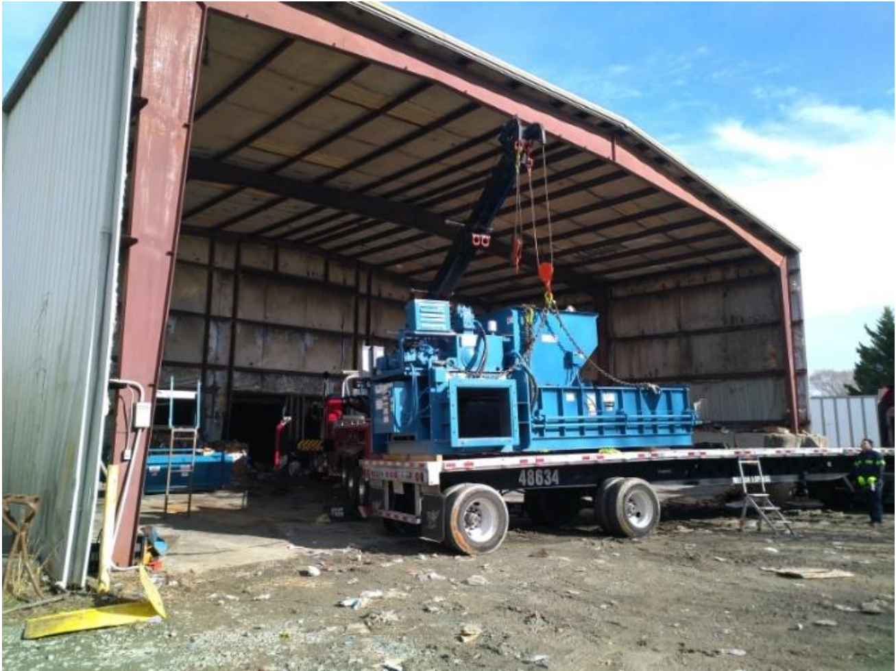
New baler in the process of being installed
