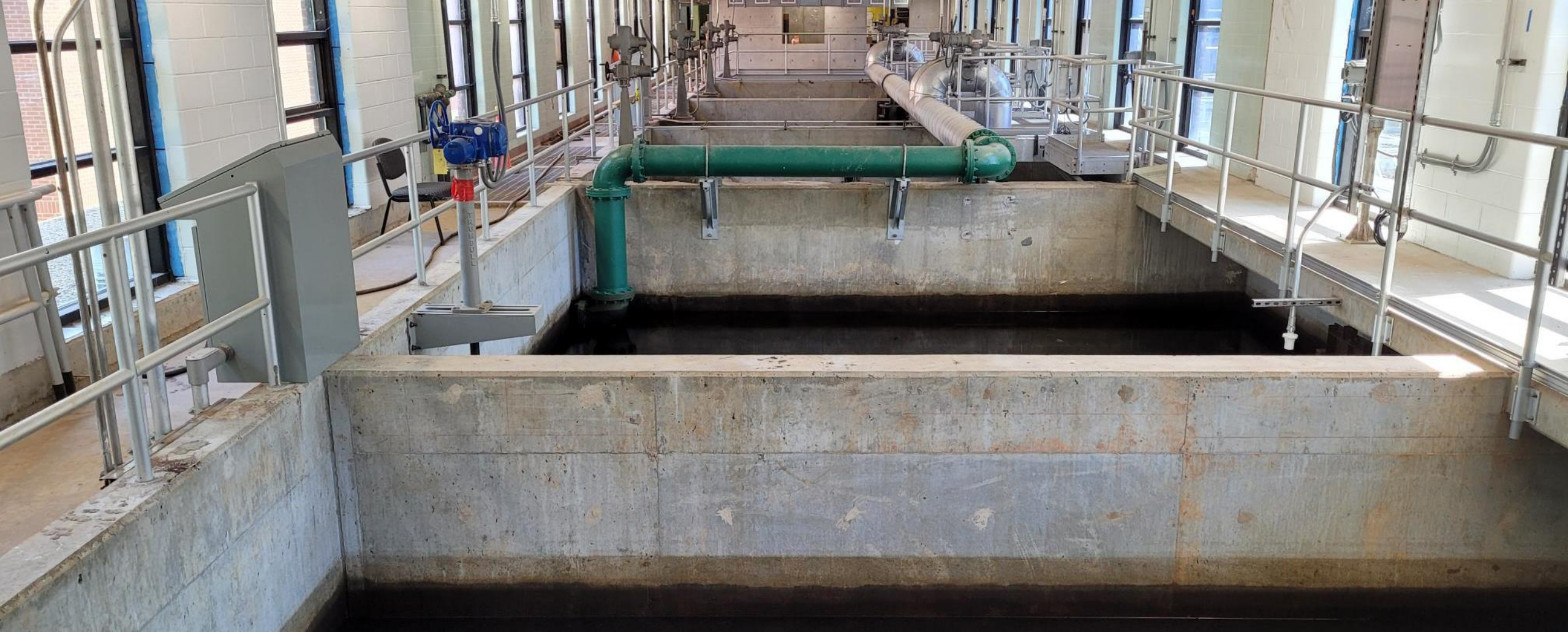
Gravity Filters at South Rivanna Water Treatment Plant
