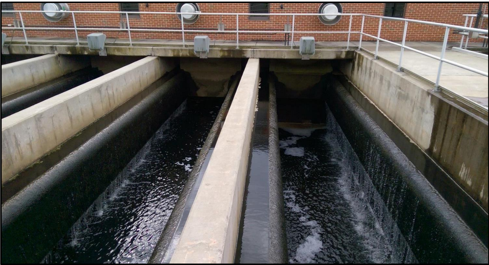
Gravity sand filters remove small particles prior to UV disinfection
