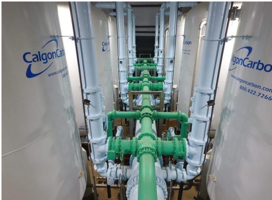
Granular Activated Carbon Vessels at the South Rivanna Water Treatment Plant
