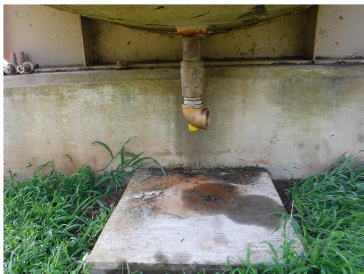
18) Drain line discharges to a concrete splash pad.
