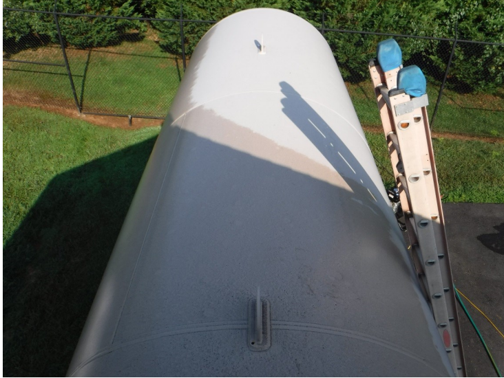
7) The coating on roof is in good condition.
