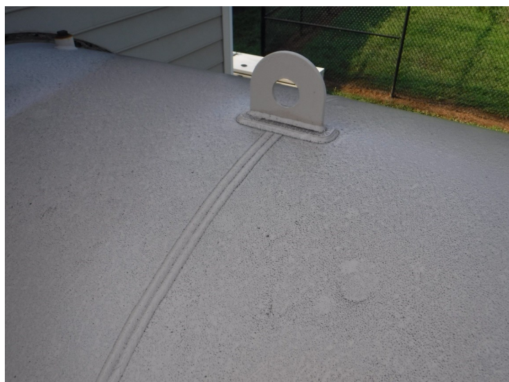
9) Original lifting lugs remain.
