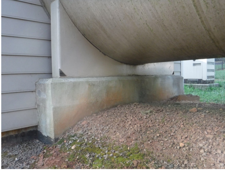
1) Coating on bottom of the tank is in good condition.
