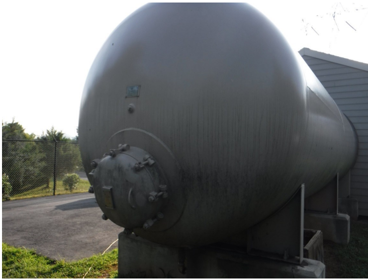
13) The coating on the exterior end cap is in good condition.
