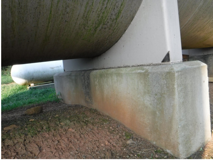
10) Concrete foundation and steel saddles are in good condition.
