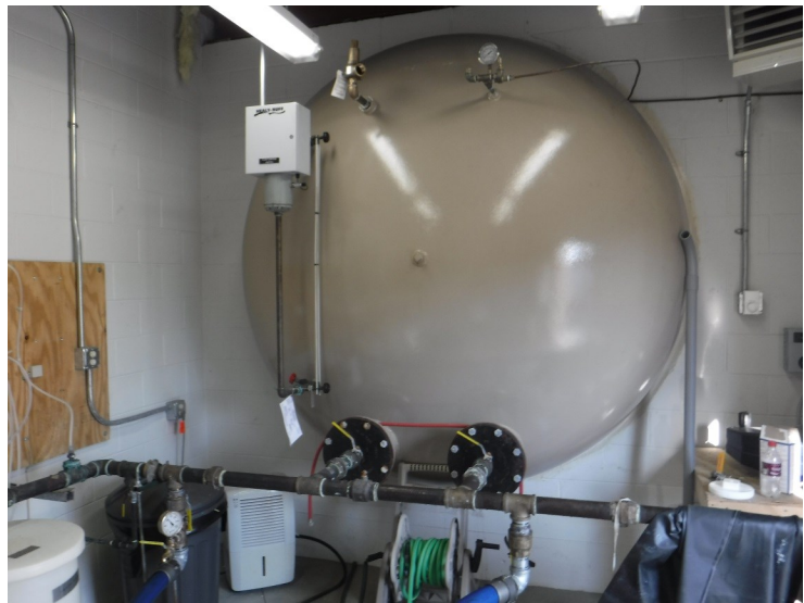
14) Interior end cap coating is in good condition.
