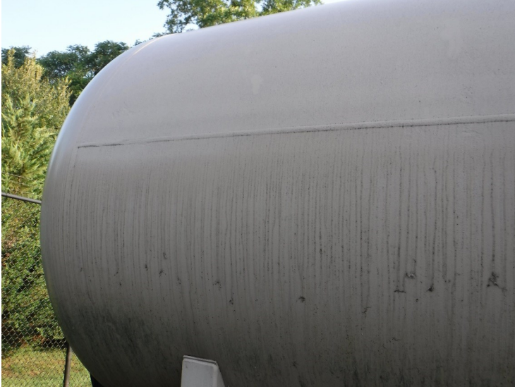
4) The sidewall coating is in good condition.
