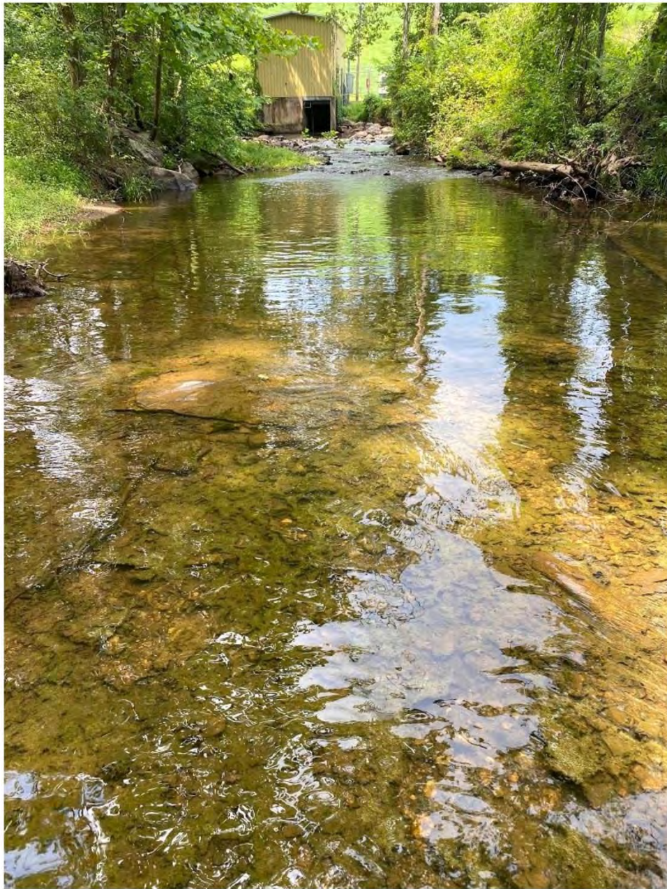
Photo 5: Beaver Creek Dam Outlet
