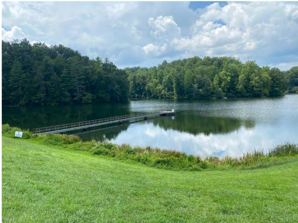
Photo 6: Beaver Creek Reservoir view from Dam
