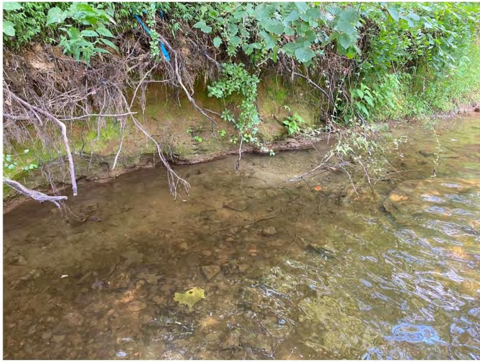
Photo 4: Beaver Creek Upper Reach Bank Scour
