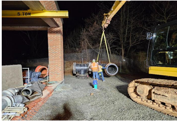
The Rivanna Maintenance team and contractors working on piping connections for the pumping bypass system.
