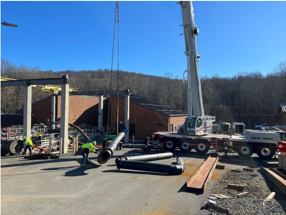
A crane lifting pipes for the bypass system
