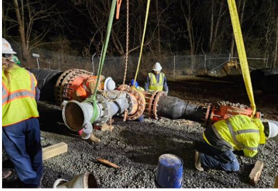
The Rivanna Maintenance team and contractors working on piping connections for the pumping bypass system.
