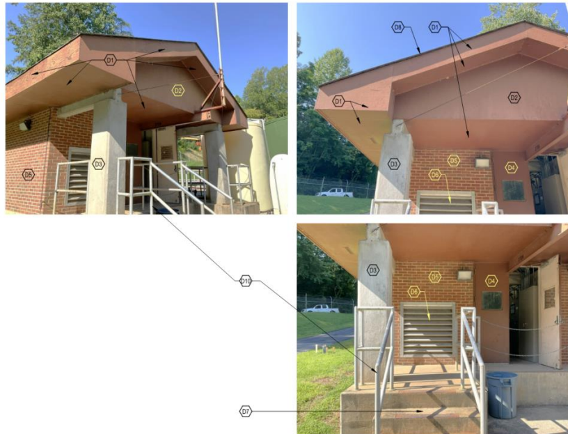
1 EXISTING CONDITIONS PHOTO FRONT OF PS4
