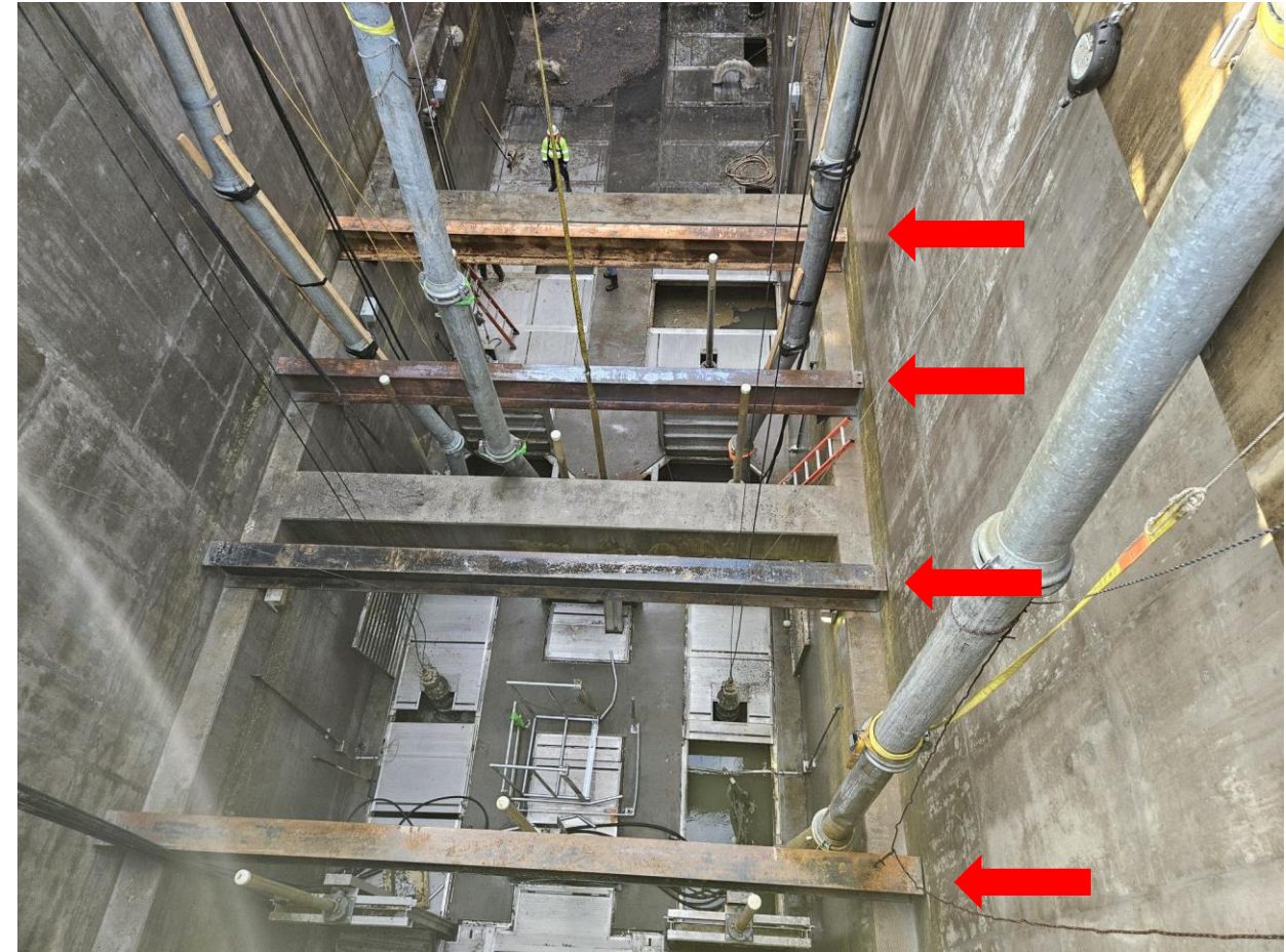
Installation of 4 Mid-Level Support Steel Beams
