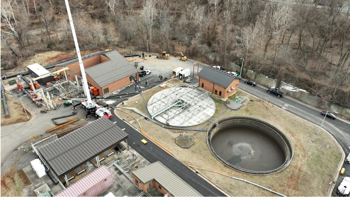
Setting up the 50 million gallon per day bypass system
