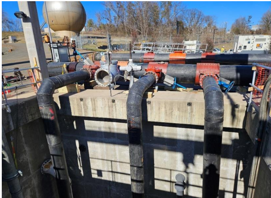
50 million gallons per day bypass under construction
