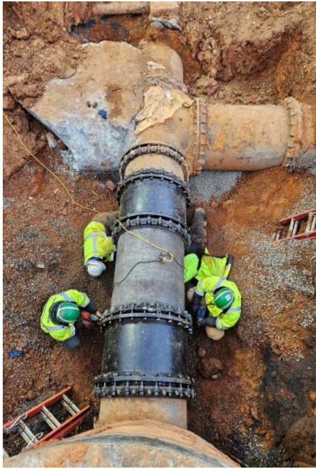
The Rivanna Maintenance team and contractors working on piping connections for the pumping bypass system.
