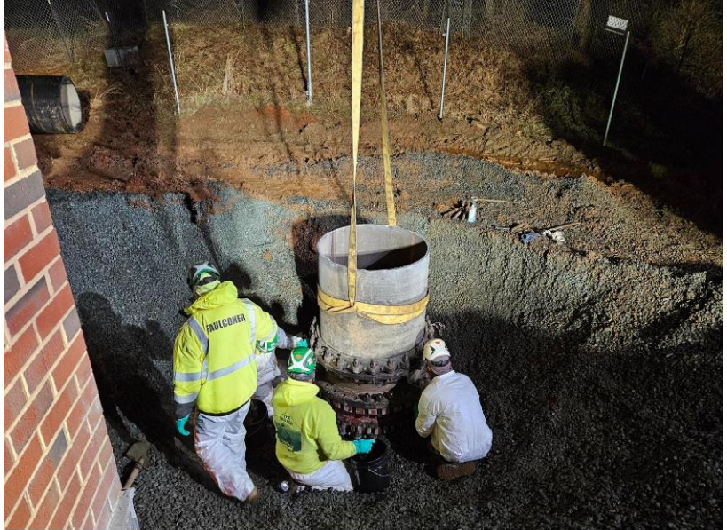
The Rivanna Maintenance team and contractors working on piping connections for the pumping bypass system.
