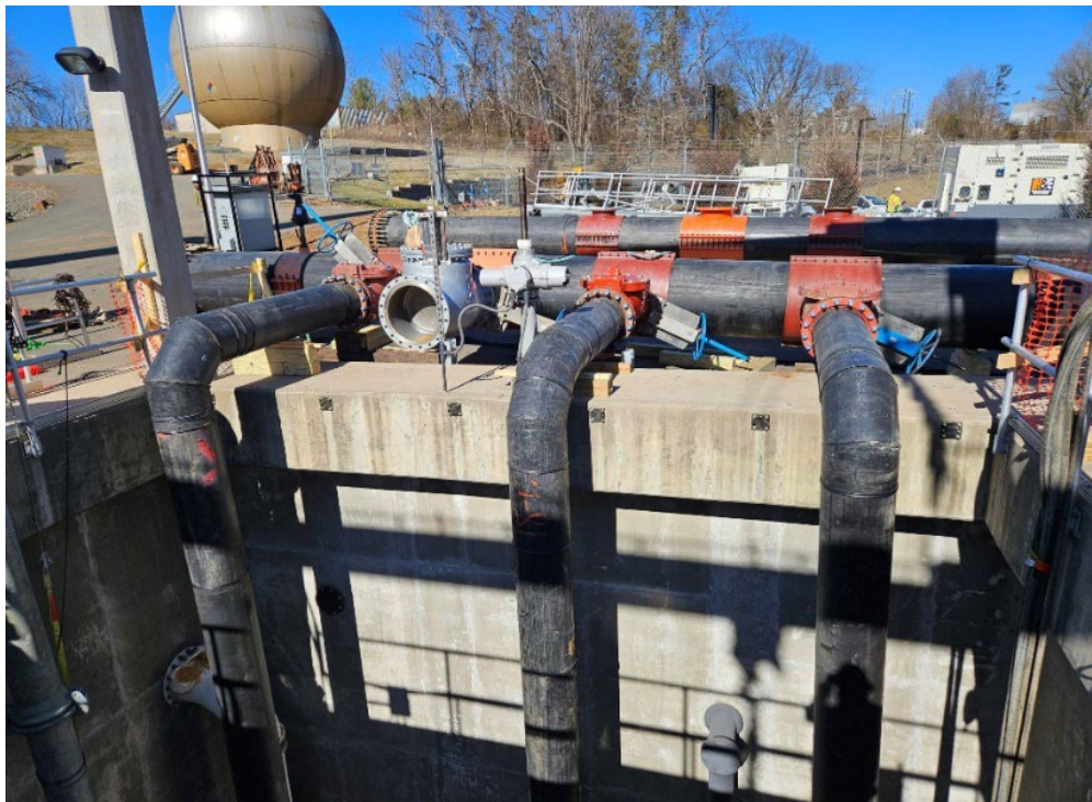
53 million gallons per day bypass under construction
