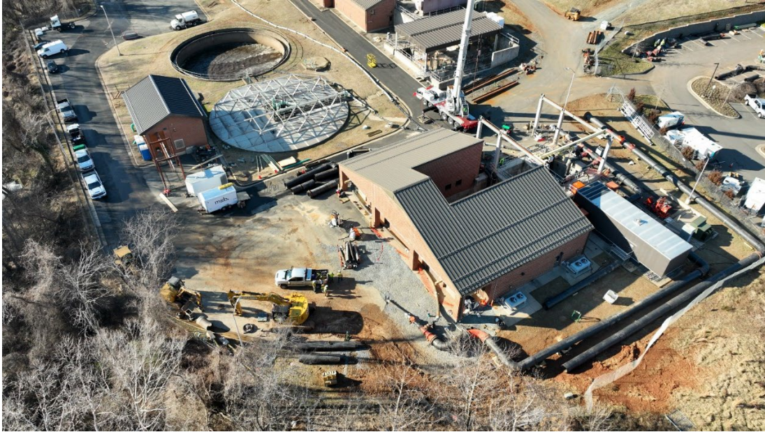
Rivanna Pump Station
