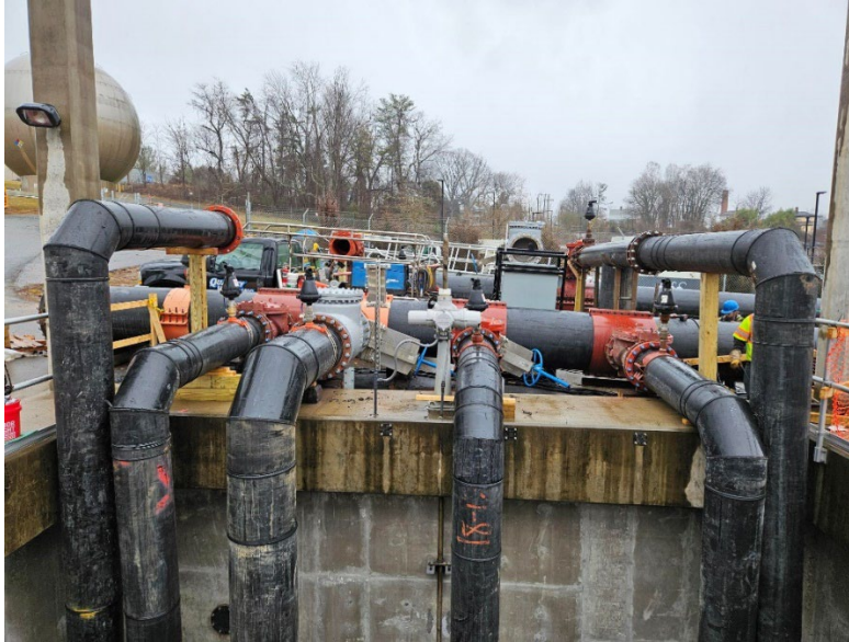
53 million gallons per day bypass pumping system
