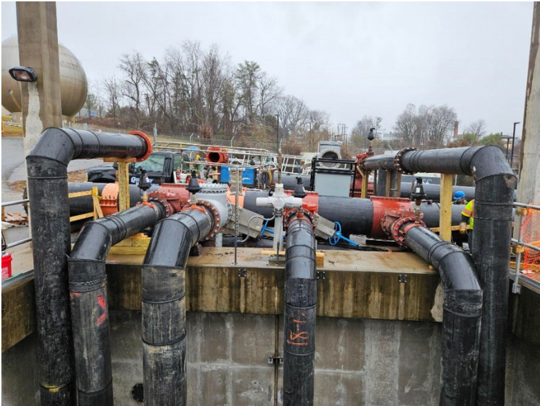
55 million gallons per day bypass pumping system
