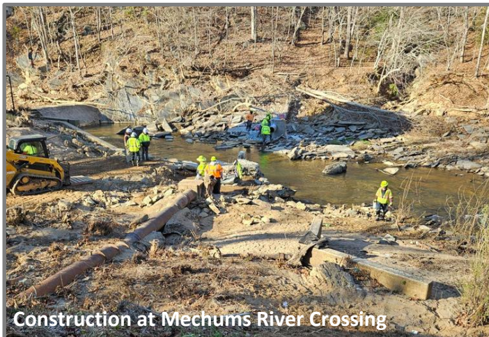
18" Replacement pipe on-site before installation
