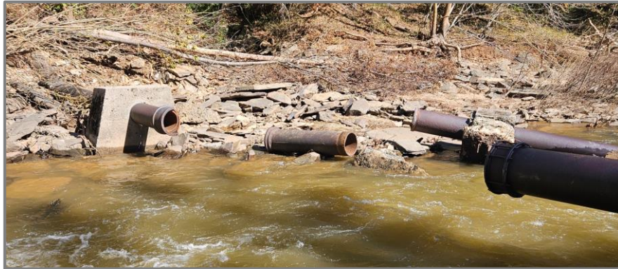
Sugar Hollow Water Line at the Mechums River Crossing damaged by Hurricane Helene
